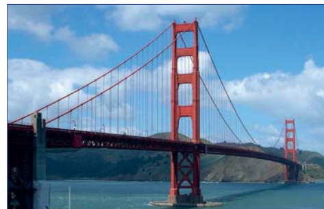
San Francisco, Golden Gate Bridge
